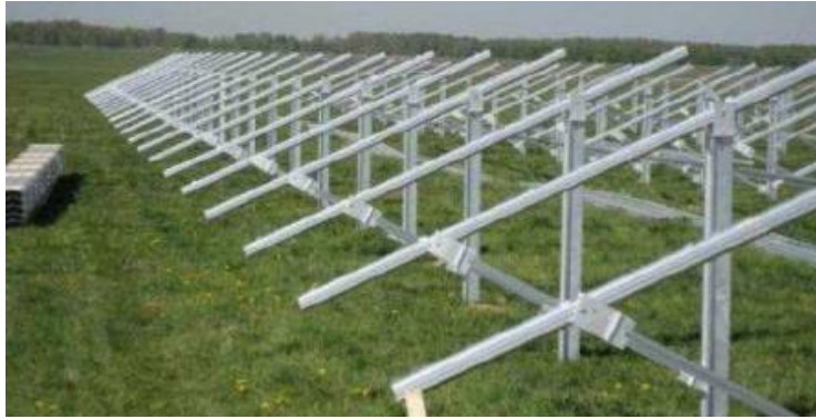
Photo 1 : Structures de support sans modules
